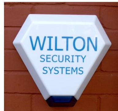
A high-intensity flashing xenon strobe is also incorporated in the external sounder. This will flash in conjunction with the audible alarm thus enabling easy identification of your premises if your neighbours have similar alarms. The strobe will also continue to flash, after the audible warning has reset, thus providing continued indication of an alarm condition at your premises without infringing noise abatement regulations. (*Clean Neighbourhoods and Environment Act 2005*)
